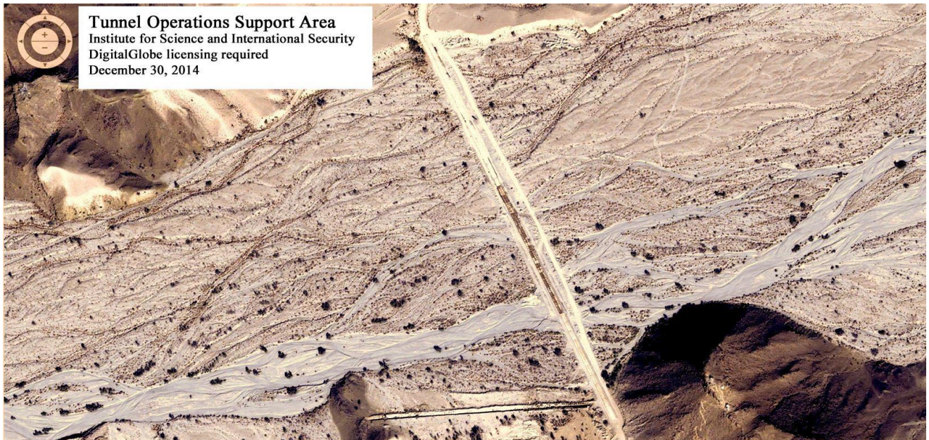
Figure 14. The access road to the Support area and the underground complex from the main highway is being covered while an alternate road is built next to the original one. This construction appears to be designed in response to the potential intermittent flooding that can be expected in this river bed. A new possible security trench can also be seen in the lower, center part of the figure.
