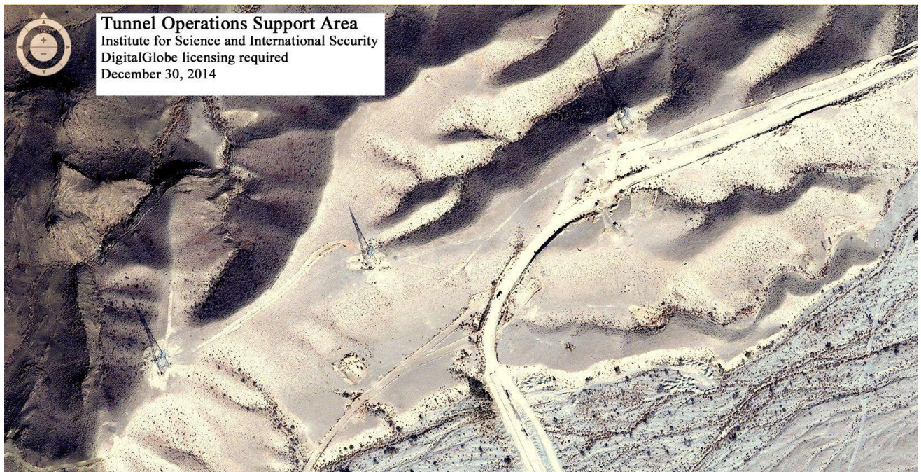
Figure 13. High power transmission line towers are visible near the road entrance to the Support area and underground complex.
