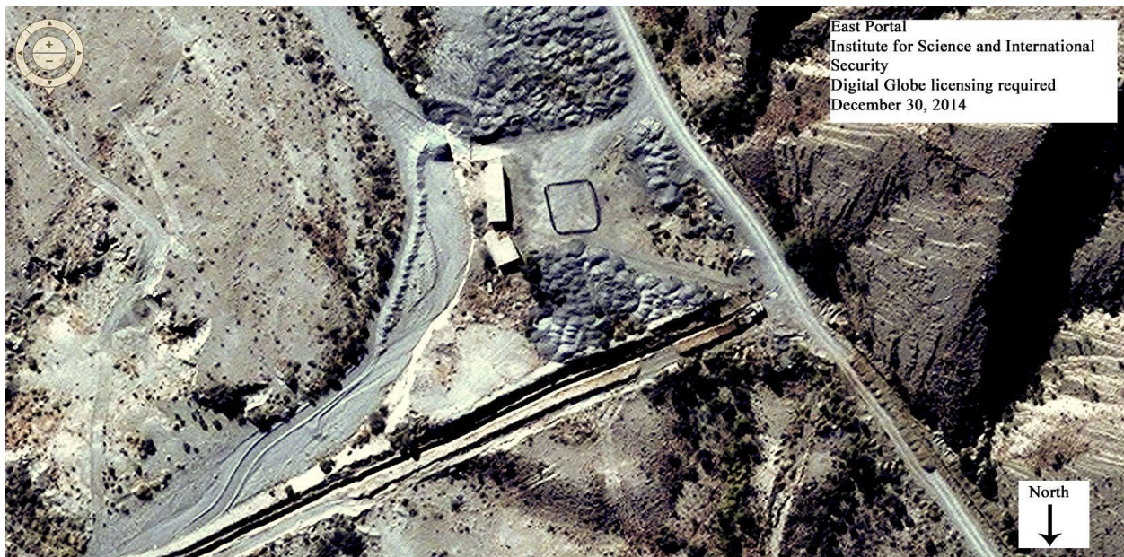
Figure 23. Approach to East portal in close-up.
